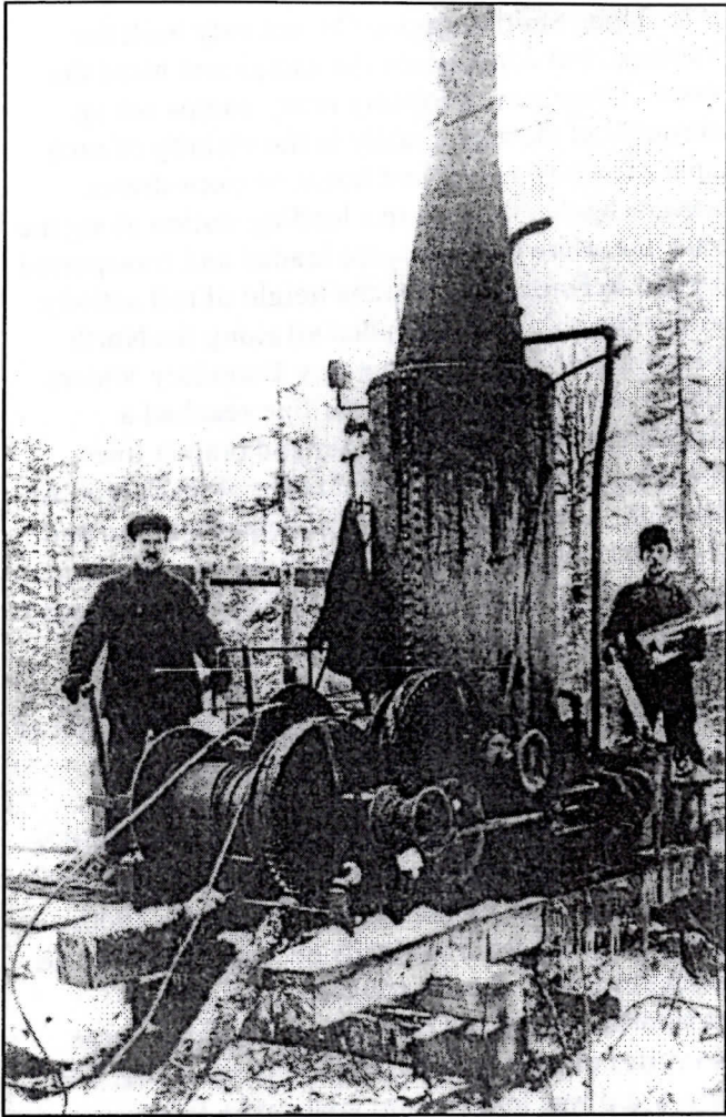
"Donkey" steam engine used for hoisting logs along the Alger-Smith Line
